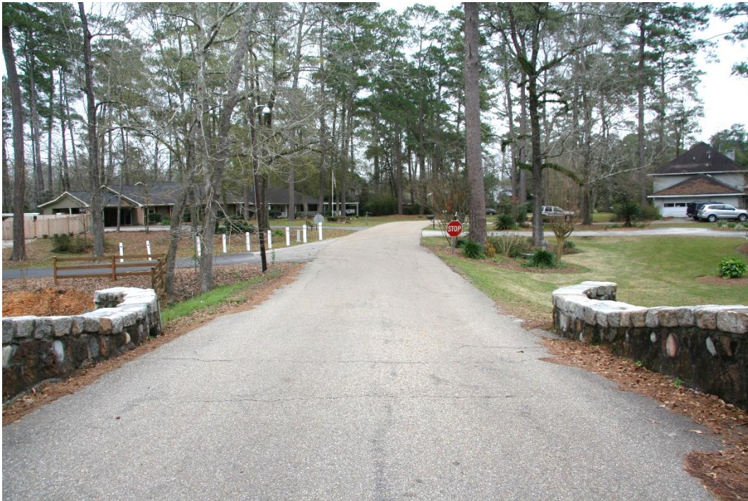
Condition Photo 2: East roadway approach to bridge, looking east.
