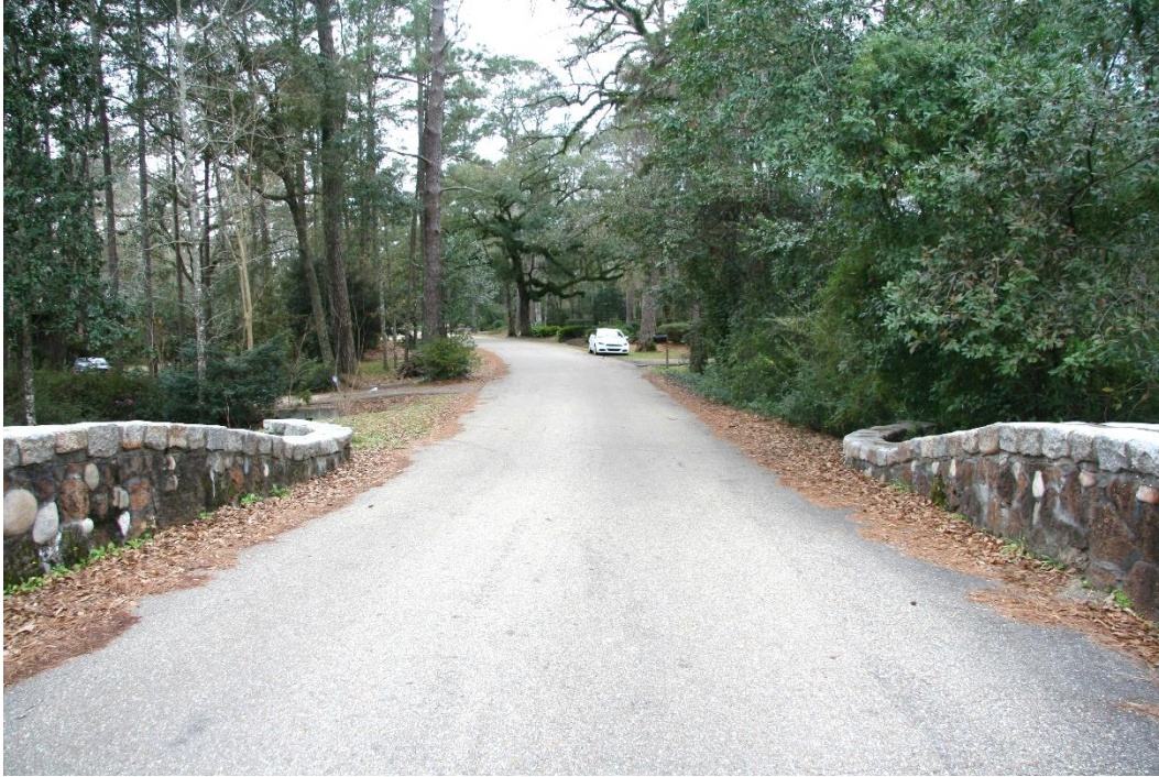
Condition Photo 3: West roadway approach to bridge, looking west.
