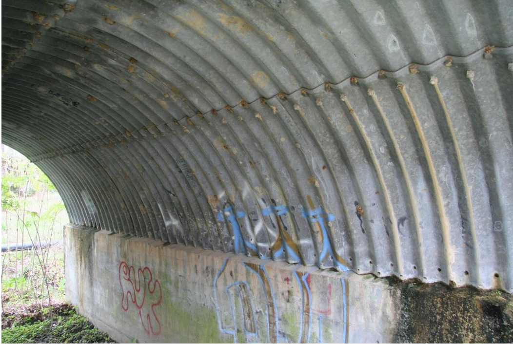
Condition Photo 9: Condition of metal liner plate detail.
