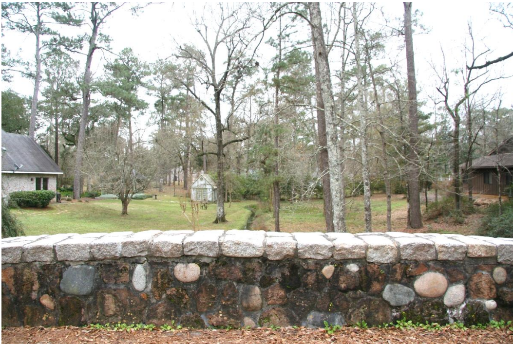
Condition Photo 4: Bridge parapet railing with capstones, looking south (upstream).
