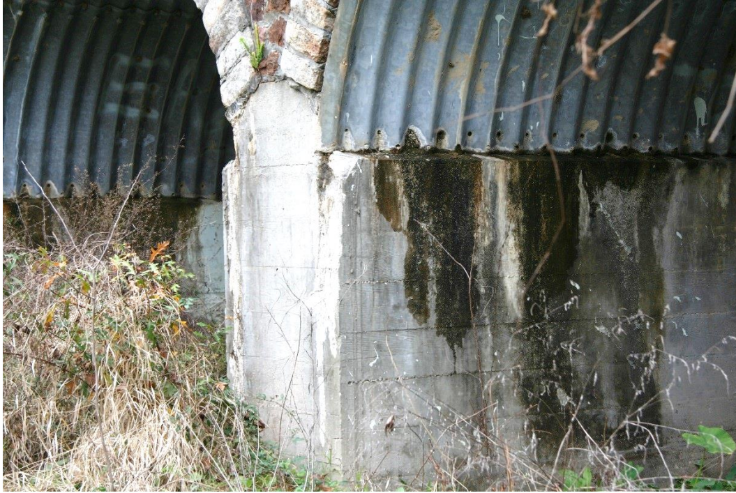
Historic Fabric Photo 1: Cast-in-place concrete foundations.
