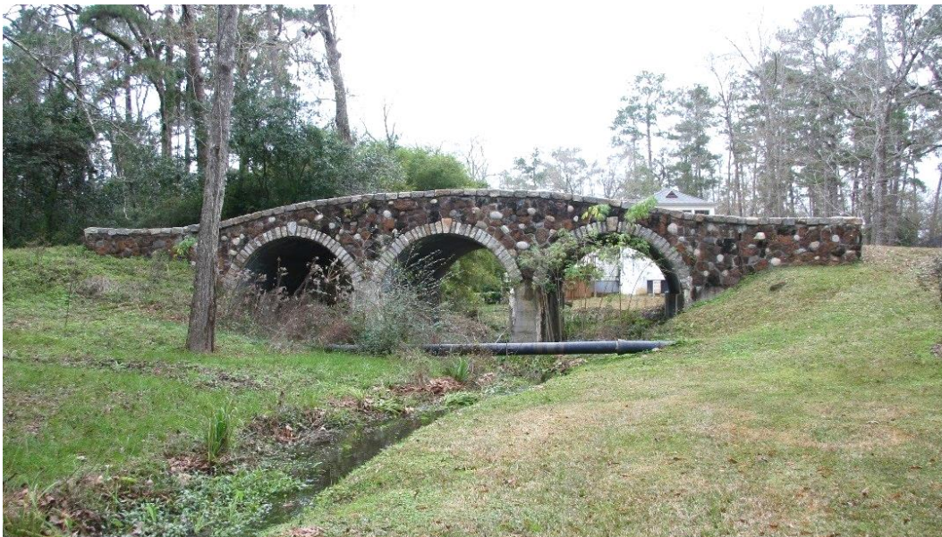
Character-defining Feature Photo 2: Ornamental mortared stonework and curved parapet railings with capstones that contribute to its high artistic value.
